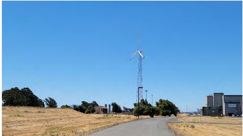
Photograph 2-8 View Looking South at Project Site and Existing Windmills
