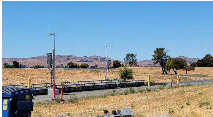
Photograph 2-5 Existing Truck Scale
