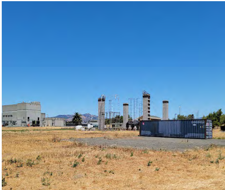
Photograph 2-7 View of Project Site and Dewatering Building looking Northeast
