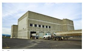
**I. Dewatering** The digested solids are pumped to the dewatering building or solar drying beds, where excess water is removed.
