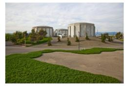
**C. Intermediate Treatment** The oxidation towers and intermediary clarifiers remove soluble organic matter.
