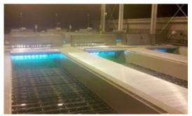
**F. Ultraviolet Disinfection (UV)** UV light destroys the genetic makeup of pathogenic organisms to prevent the spread of waterborne diseases to downstream users and the environment.
