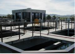
**E.** Tertiary Treatment Filters provide a polishing step to remove the few suspended particles remaining in the secondary clarifier effluent.
