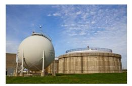
**H. Anaerobic Digestion** Solids removed in the clarifiers are thickened and then digested in a closed vessel. Digesters provide an environment to reduce the organic matter and disease-causing organisms. Methane is produced as the solids are digested and is used as a fuel for on-site electrical generators.
