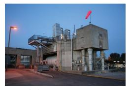
**A. Preliminary Treatment** Debris and grit that are harmful to downstream equipment are removed with bar screens and degritting equipment. Influent flow is measured and recorded at this location.
